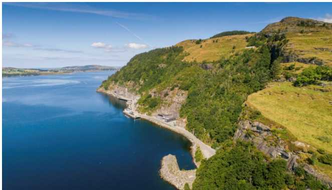
Green Mountain's SVG1-Rennesøy data center
